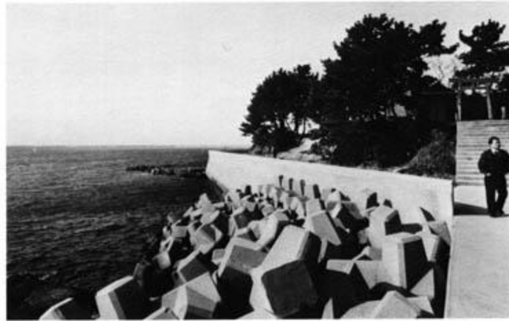
The natural shoreline has disappeared under concrete tetrapods at Cape Hiruko, Kira.
